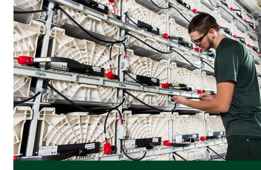
Based on your power and space requirements, an Eos Cube project can range from a single to a multi-Cube installation. A single-stacked Cube installation rated at 10MW/40MWh requires approximately 25,000 square feet.
