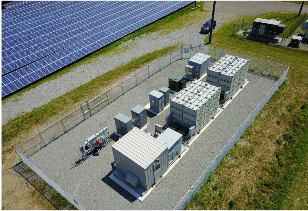
1 MWH GRID-CONNECTED SOLAR + STORAGE + DIESEL MICROGRID AT PSE&G SITE
